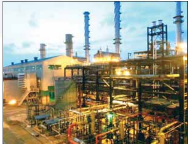
Captive Power Plant
