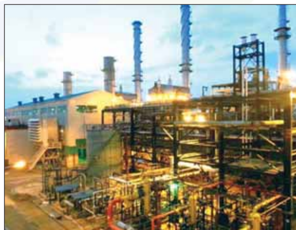
Captive Power Plant
