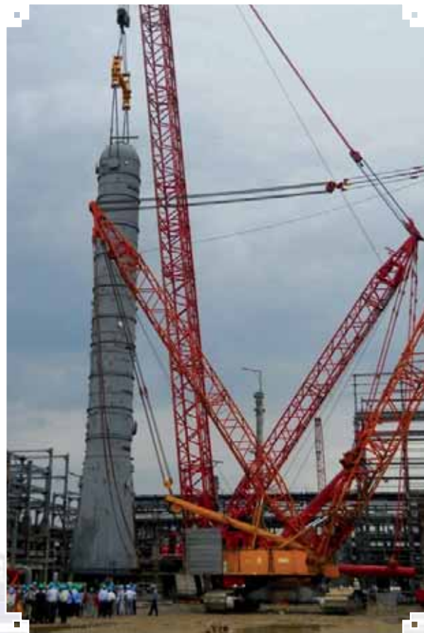
Erection of the Gasoline Fractionator in the Ethylene Cracker Unit.
