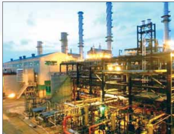
Captive Power Plant
