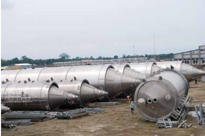
Cyls for the HDPE/LLDPE unit
