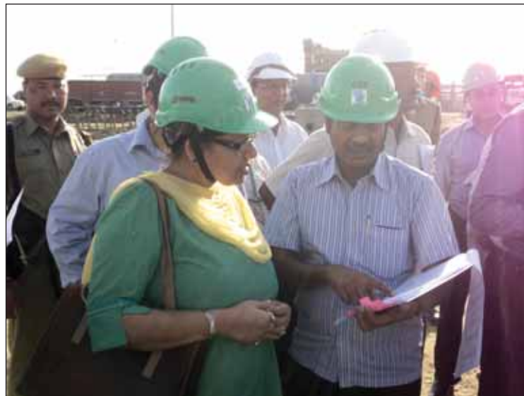
Reviewing progress : The Joint Secretary, MoCF, Ms Neel Kamal Darbari with the Chief Operating Officer, Shri P N Prasad at Lepetkata
